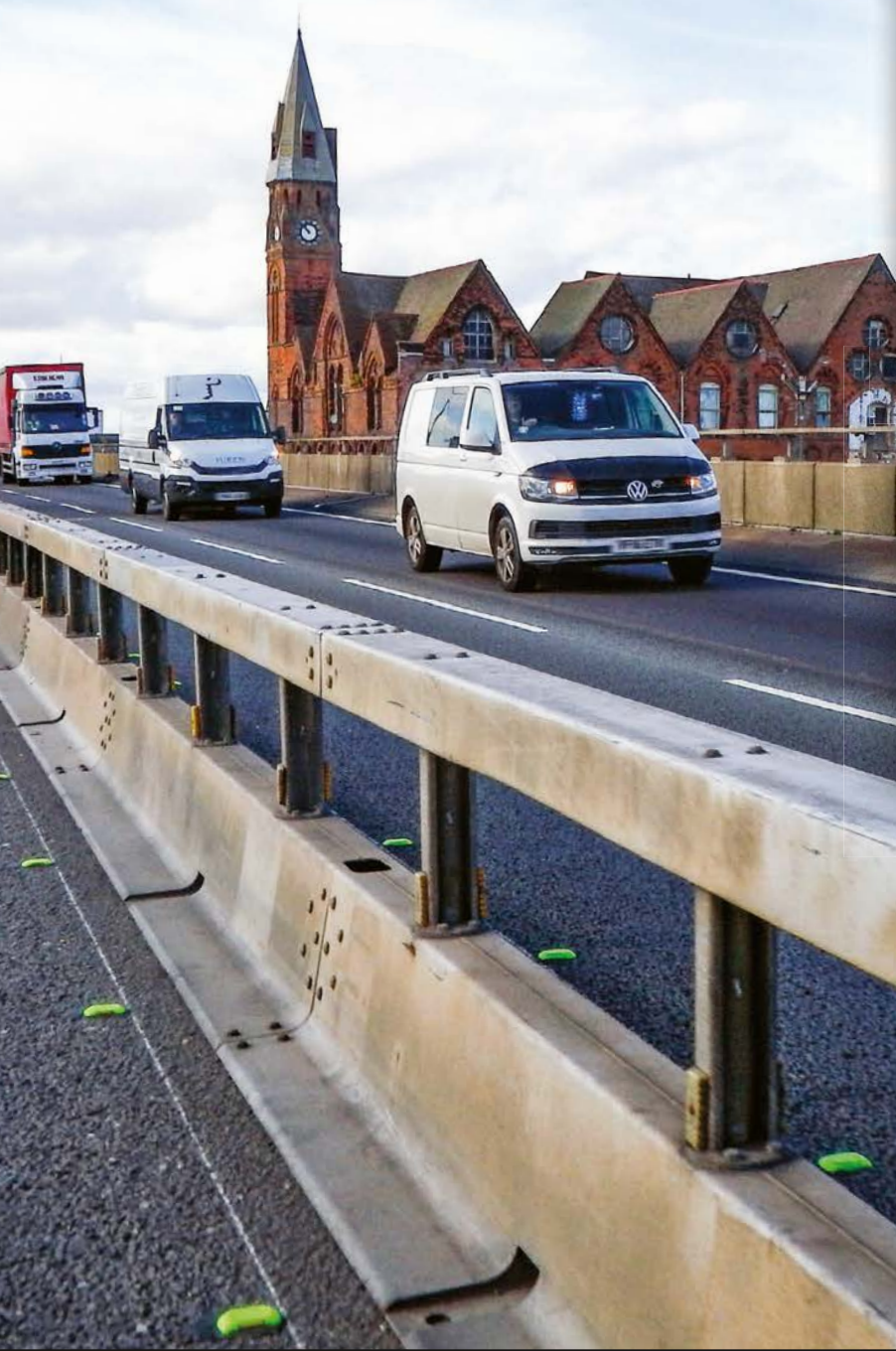
Image: Asset Varioguard with Concrete Mass Anchor System, M5, Jct 1 - 2, Oldbury
