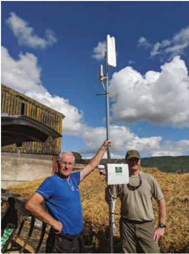
Antenna installer Ian Newman and Ch4Ike champion Nick Birkett preparing a 4G cell to be mounted on a barn at Rookhay Farm. The complete installation (which included the wireless meshing equipment) was set up on a single aluminium pole, which was then bolted to the steel structure of the barn.
