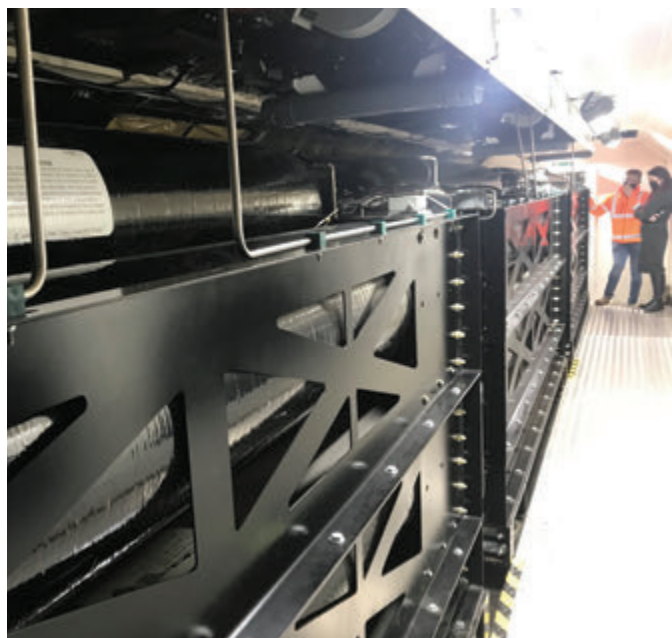
The hydro chamber features three banks of 12 hydrogen fuel cell tanks for a total of 36 150kg tanks, with total capacity for 277kg of green hydrogen.
