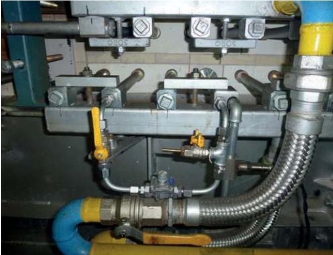
▲ Fig 2. Sorg OMT unit mounted on forehearth
